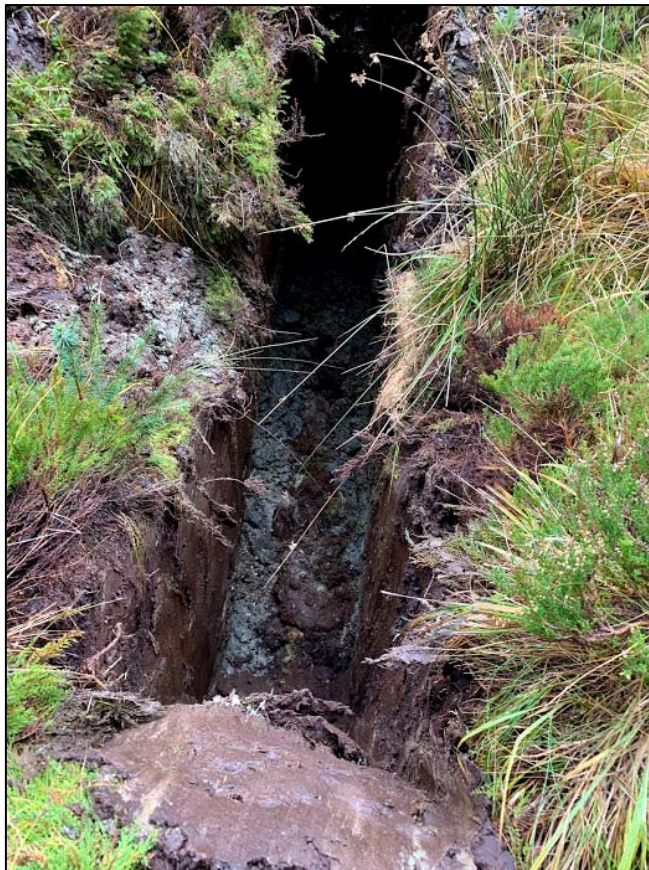
Photo 2 Trial pit T12 - TP03
