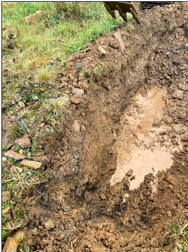
Photo 10 Trial pit BP – TP03
